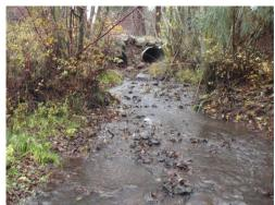
Many miles of stream are inaccessible to fish because of barrier culverts. Road culverts and other stream-crossing structures that are aging, too small, or improperly installed can block fish from reaching their spawning grounds.
